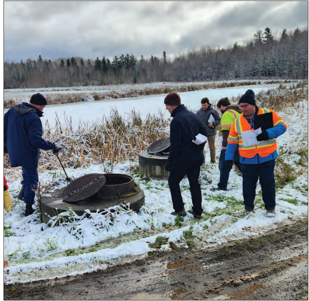
Members of the St. Paul District team met with the contractor, Indian Health Services staff and the tribal sanitation facilities supervisor at the sewer lagoon to examine existing conditions, in Nett Lake, Minnesota, Nov. 13. USACE St. Paul District courtesy photo
