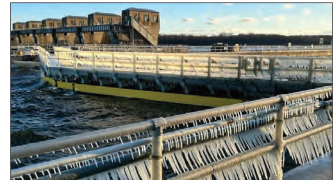
Icy conditions at Lock and Dam 5 in Minnesota City, Minnesota. USACE St. Paul District photo by Judy Denzer
